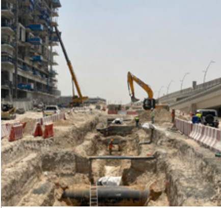
INFRASTRUCTURE & UTILITY WORKS
